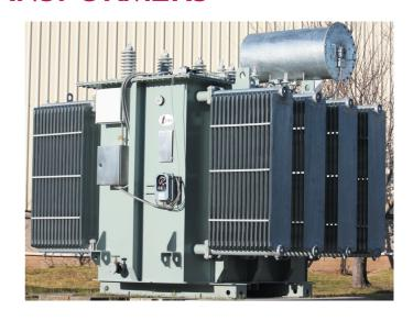
Tyree Power transformer tanks are boiler designed and fabricated, featuring Australian Standard tropical and marine rated surface treatments.
