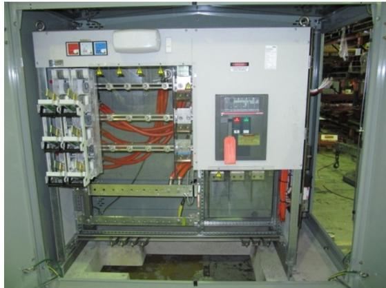
LV board with isolator, provision for fuse strips, generator connection point and C/B.
