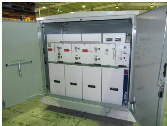
EFACEC HV switchgear. 11/22kV SF6 unit with 3 switch functions and 1 fused transformer function
